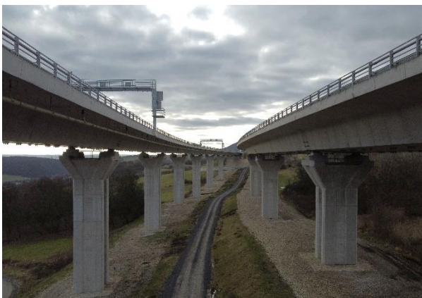
Figure 8. A view of the investigated viaduct.
